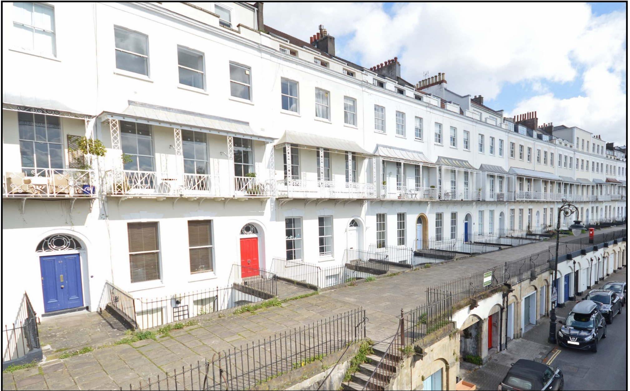
TOP FLOOR FLAT, 5 ROYAL YORK CRESCENT, CLIFTON, BRISTOL, BS8 4JZ
